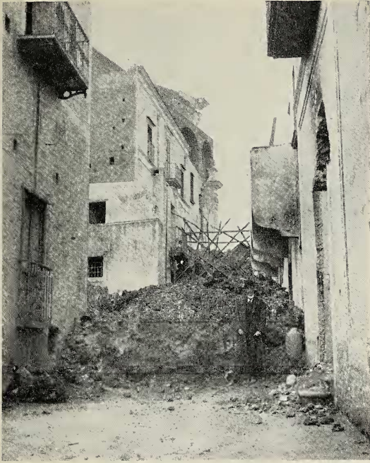
FIG. 3. Lava flow filling a street in the village of Boscotrecase on the slope of Vesuvius during the eruption of 1906. Note that the masonry walls are little disturbed. Photo by T. A. Jaggar.
